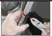
After pulling the zip ties as tightly as possible by hand, use pliers to tighten all zip ties fully.
