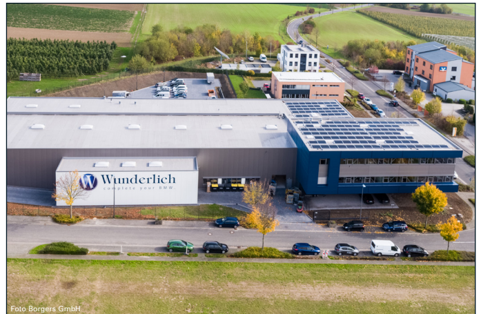
Foto Borgers GmbH The Wunderlich company headquarters in Graftschaff-Ringen
